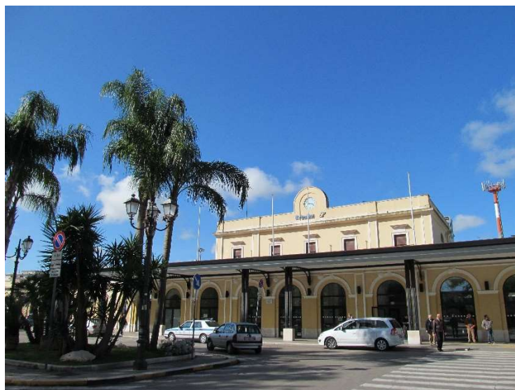
Brindisi Rail Station
