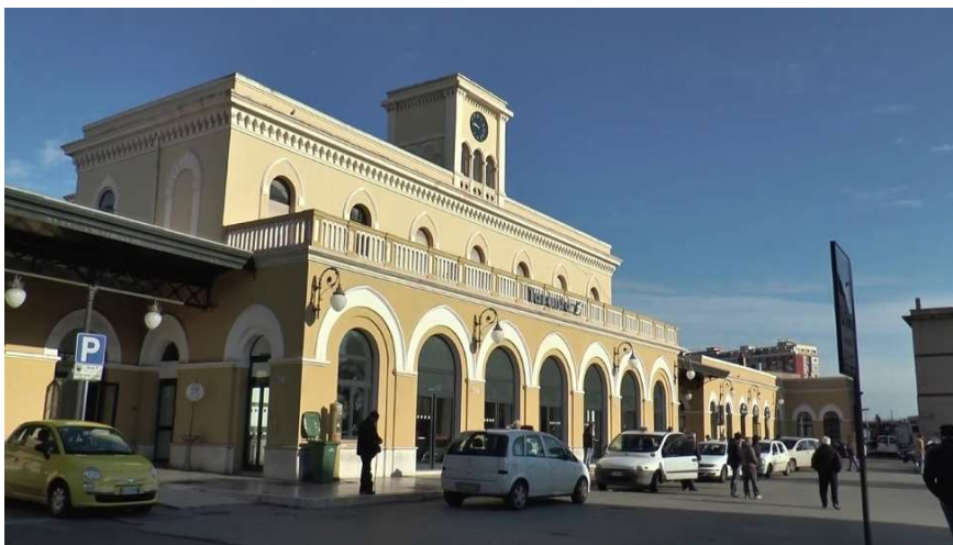
Taranto Rail Station
